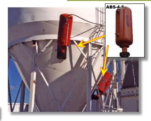
A customer was having problems with oak and maple sawdust would bridge above the unloader whip. This caused production to be halted and some one had to hit the silo with their head.
