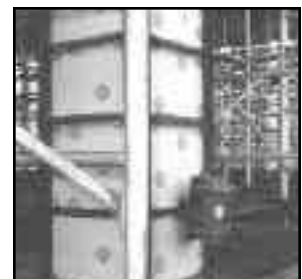
US-1600 with "Clamp-On" bracket on wooden form with steel reinforcing
