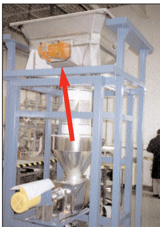
SCR-300 on Box Dumper to prevent hang-ups.
