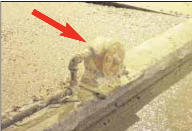
VS-510 SILENT TURBINE VIBRATOR ON CONCRETE SCREED eliminated blemishes from ball vibrator lubricant leaks and reduced noise levels significantly.
